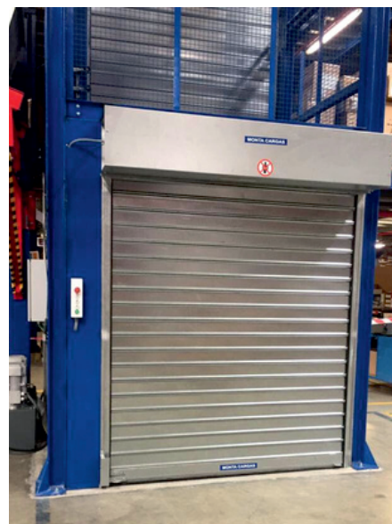
Porta Grade de Enrolar em Chapa Lisa Smooth Plate Rolling Grid Door
